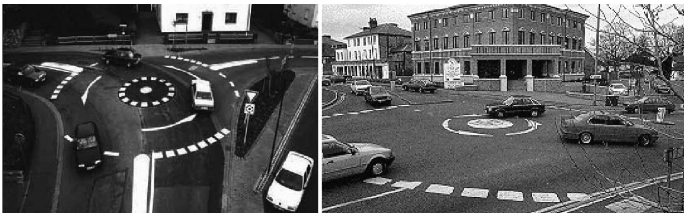
Figura 5 - Mini-rotundas (fonte FHWA, 2000 e Public Roads, Autumn 1995, Vol 59, Nº2)
