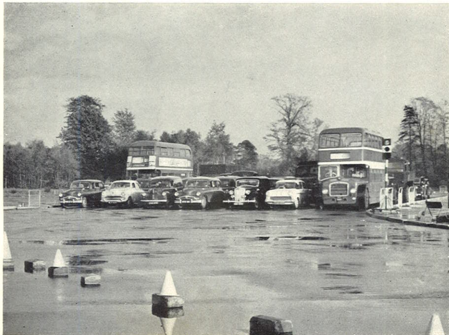
A 60-ft wide approach used in a controlled experiment on traffic capacity PLATE 4
