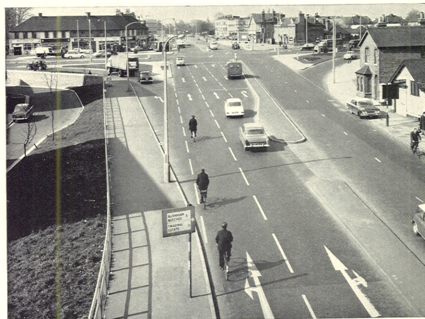
Double right-turning lanes at an intersection in Slough, Bucks
