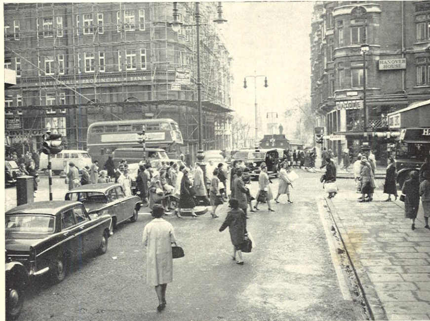
A typical 'poor' site PLATE 8
